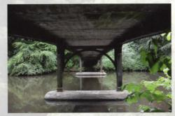
deck comprises twin steel fabricated girders, connected transversely by steel rolled beams encased in a concrete slab. The slab is surfaced with tar macadam. The deck is supported on concrete abutments and cast iron intermediate column supports, linked transversely by elegantly curved cast iron cross bracing. The columns are connected by sole plates to concrete foundations, which also act as "cutwaters". Decorative cast iron parapets complete the structure.
